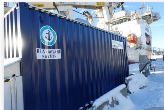
Bilde 4: Mobil 20' landstrømcontainer
